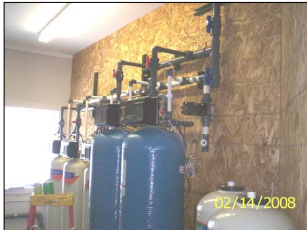
Modular AD26 Oxidation/Filtration and E33 Adsorption System
