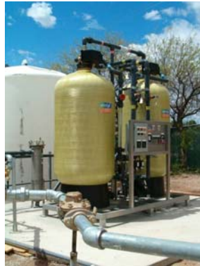
After Installation May, 2004
