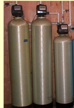
Modular with Composite Tanks
